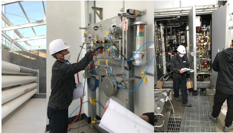
Site review, inspection and regulatory coordination remain part of practical readiness
